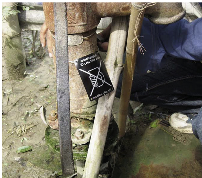
Fig. 1. Tube well and test result plate. The picture shows an example of the black-and-white plate used to communicate results: the plate indicates the well I.D., the year when the water sample was taken, the arsenic level and a hand holding a drinking cup, in this example crossed out because the arsenic level (336 ppb) is above the safety threshold. The smaller, stainless steel plate visible above the black-and-white one indicates the well I.D. and was attached to the well in 2005, at the time of the water sample collection.
